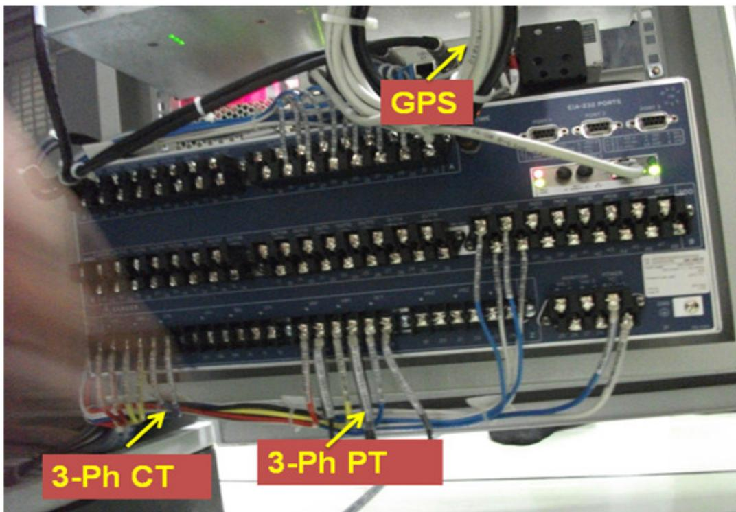
Figure 11: Inputs to Phasor Measurement Unit
