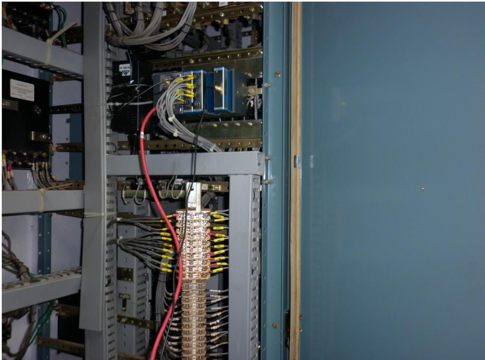
Figure 31: Installed PMU at Raipur
